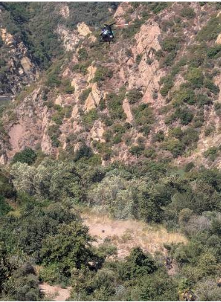
Picture Caption: With Malibu Canyon's narrow and severely limited access, a Boeing CH-47 Chinook helicopter was needed to transport special equipment into the dam site to conduct Geotech studies. Among the supplies air dropped in were a drill rig, small excavator, front end loader, metal bridge, side-by-side ATV, tools and other supplies.
